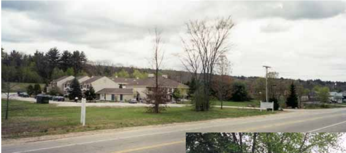
City of Franklin – Franklin Plantation
