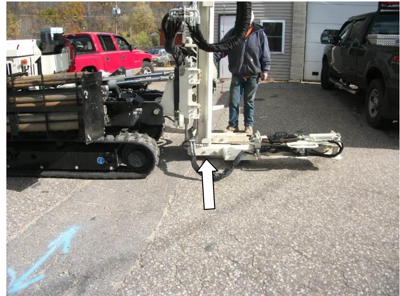
6. Location of CA-SS-2 to west of Site building facing east
