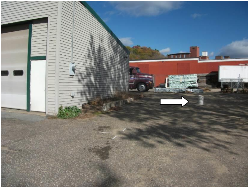
7. Location of CA-SS-1 to south of Site building facing east
