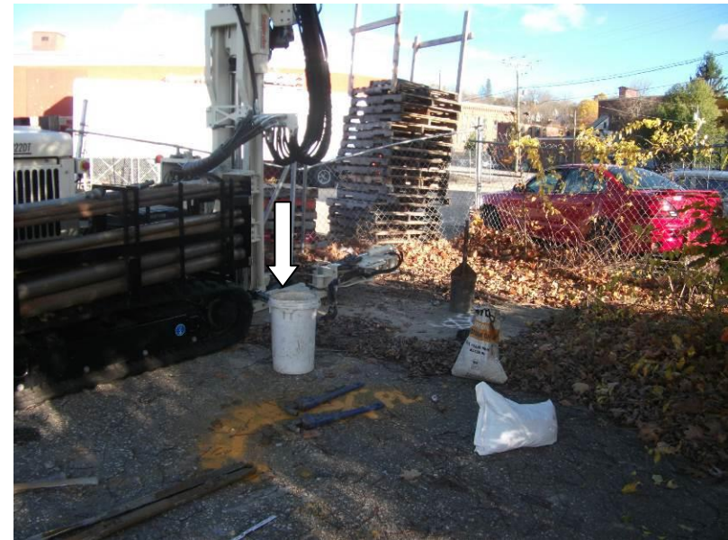
4. Location of CA-SB-4/CA-MW-4 to southeast of Site building facing east
