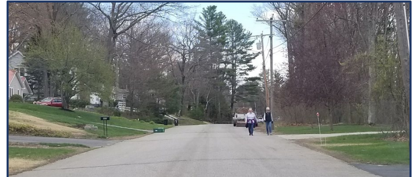
On Road – Shore Drive Paint & Signage Only
