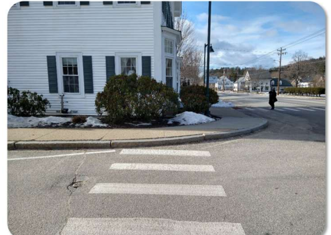
Photo 7: Non-compliant pedestrian crossing.
