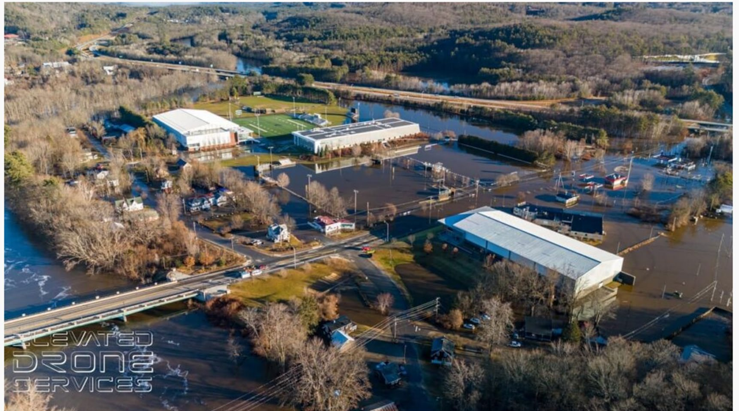
Ariel view of the flooding that occurred on 12/18 at Plymouth State University in Plymouth, NH
