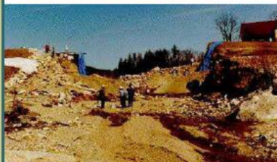
Alton dam breach, 1996
