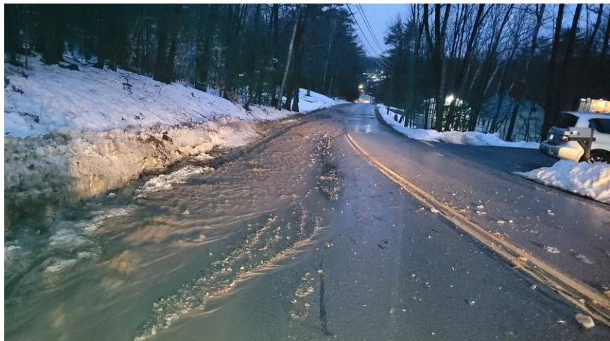
Flooding in Gilford from December 2022 Declared Disaster
