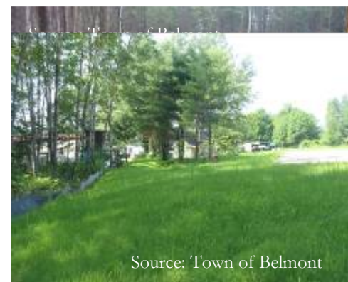
Same parking lot site after seed is established – note silt fence still up to minimize sediment runoff until complete
