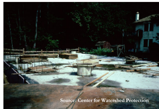
Underground sand filter during construction
