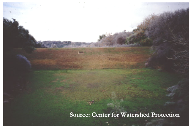
Source: Center for Watershed Protection Dry ED pond for large runoff capacity – lack of woody vegetation on embankments protects structural stability
