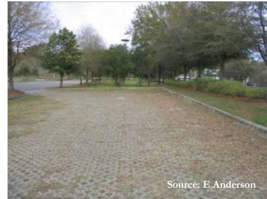
Permeable pavers for overflow parking
