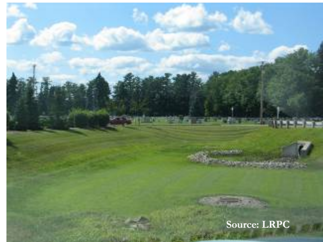
Infiltration basin for large parking area with check dam at inflow
