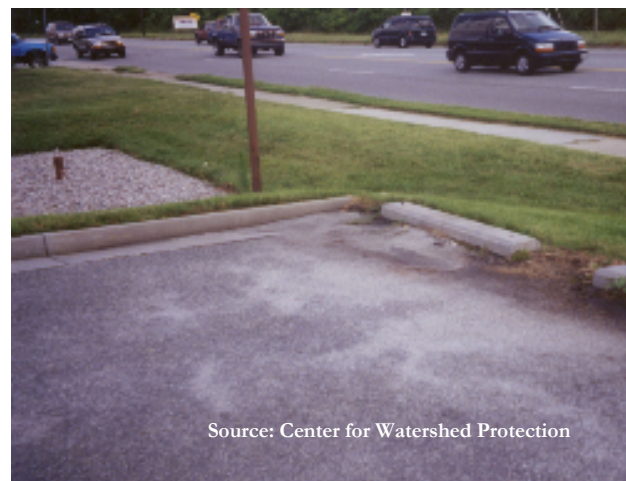
Infiltration trench next to parking lot with vegetated swale as pretreatment
