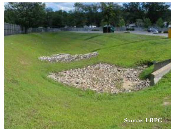
Source: LRPC Vegetated swale and check dam used as pretreatment for the infiltration trench
