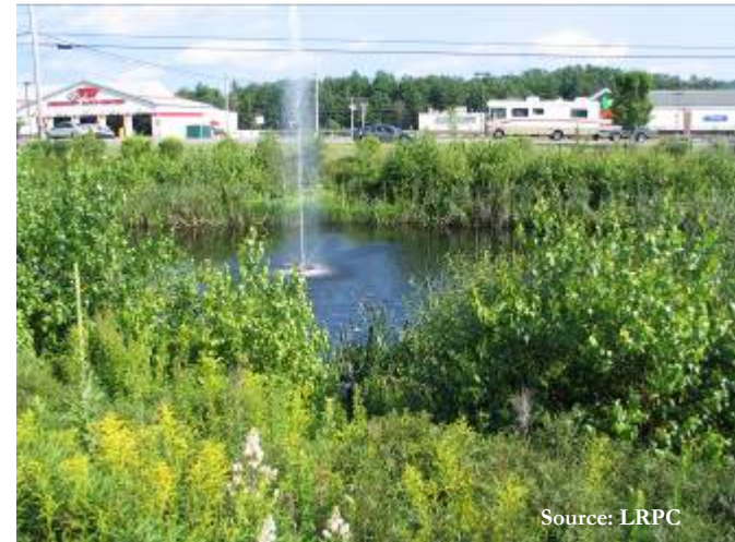
The fountain in this constructed wetland aerates water while treating parking lot runoff
