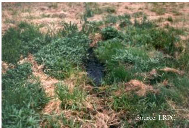
Raw sewage in a septic field from a failing system
