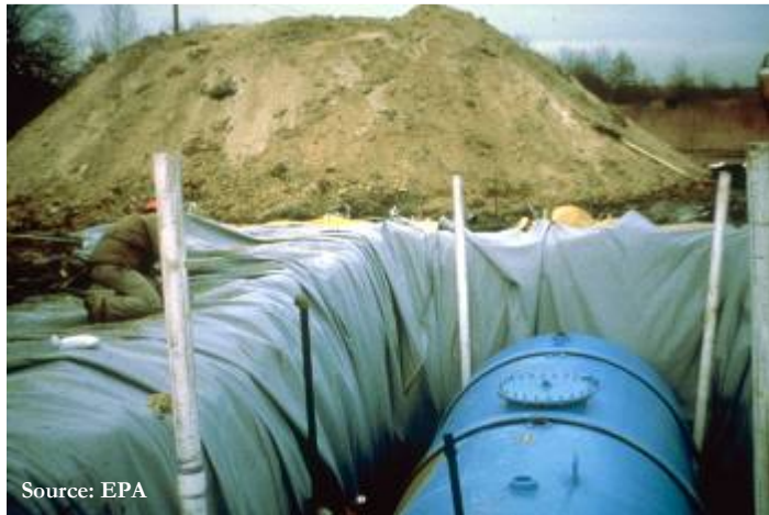
Underground storage tank in lined excavation
