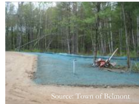
Newly seeded parking lot site – note the silt fence in the background
