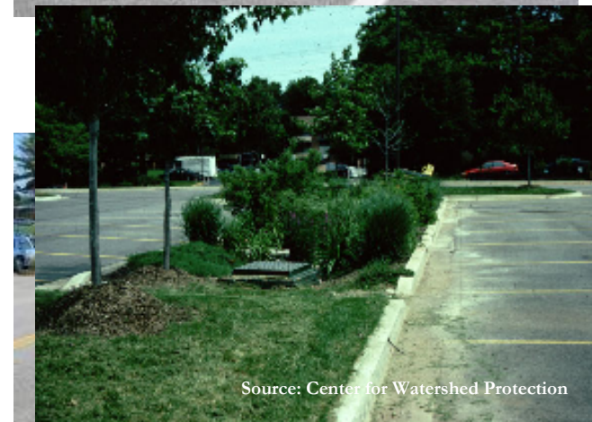
Curb cuts allow runoff to flow from the parking lot into the bioretention area.
