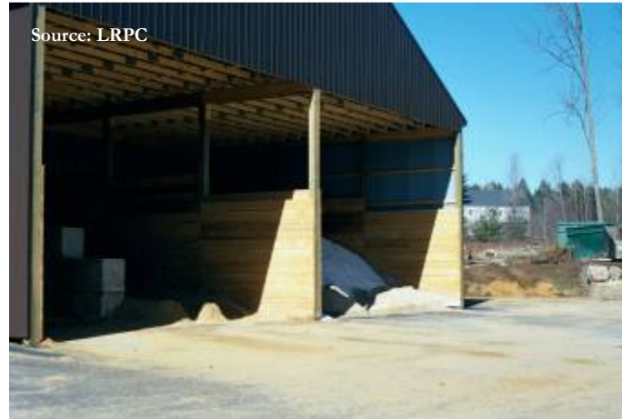
Storage facility for salt and sand
