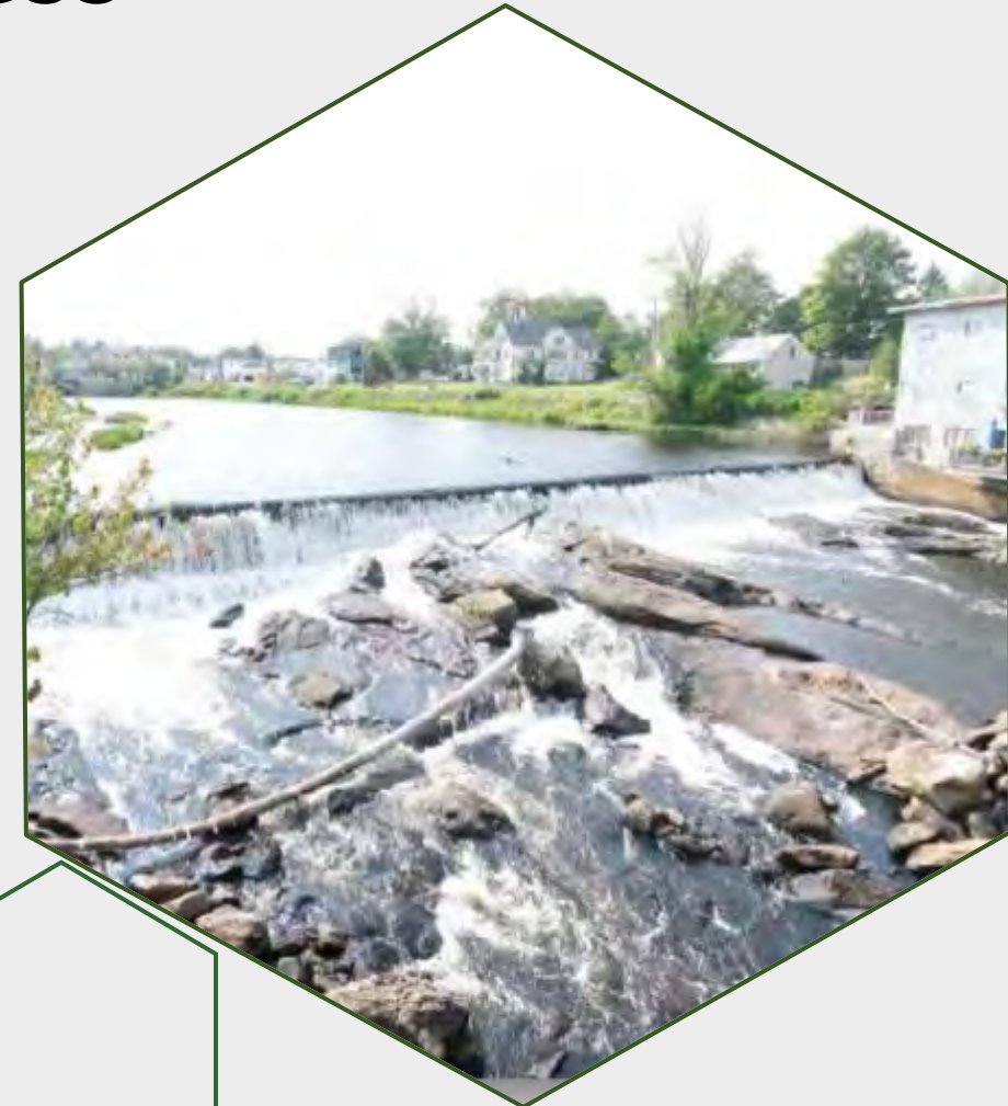
Hadley Falls Dam Removal, Merrimack River Service Area photo credit: NHDES Dam Bureau.
