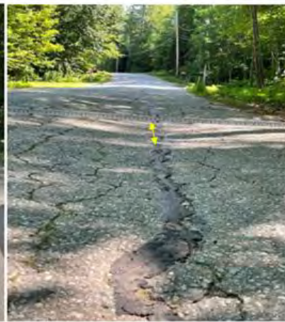
Example of rutting (note straightedge)
