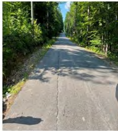
Example of longitudinal cracking
