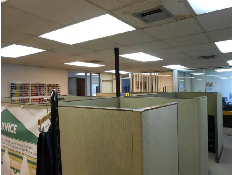
1. View of the second floor offices in the Madeira office and warehouse building.
