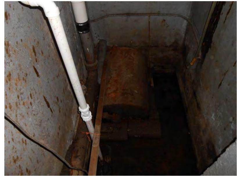
24. View of sump in the former boiler room of the two-story building.
