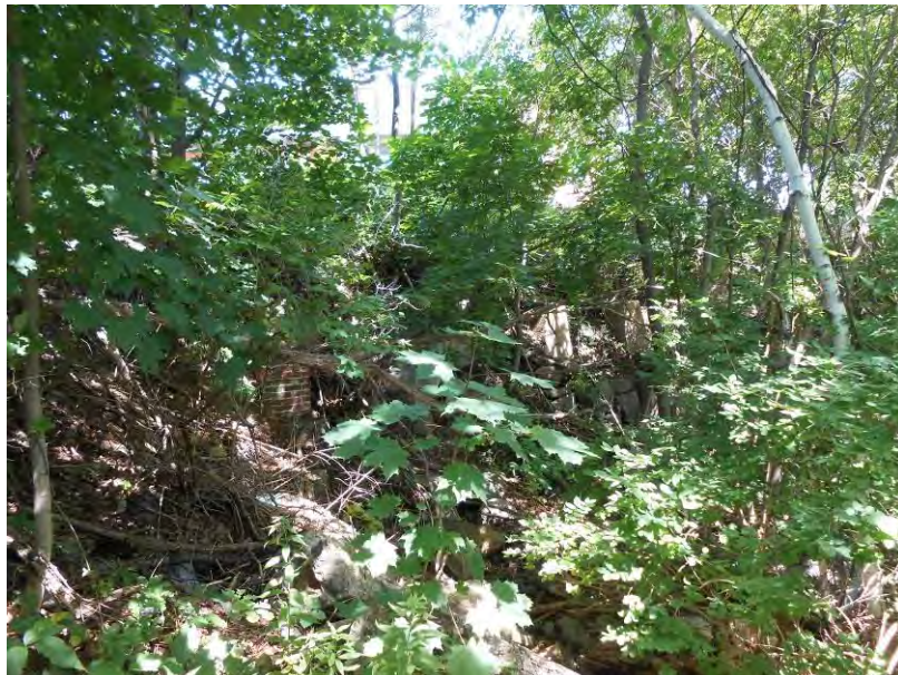
35. View of southeast portion of the Site which was overgrown with vegetation. Foundations and fill were observed.
