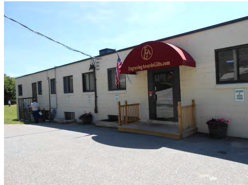
16. View of the entrance to the two-story building.
