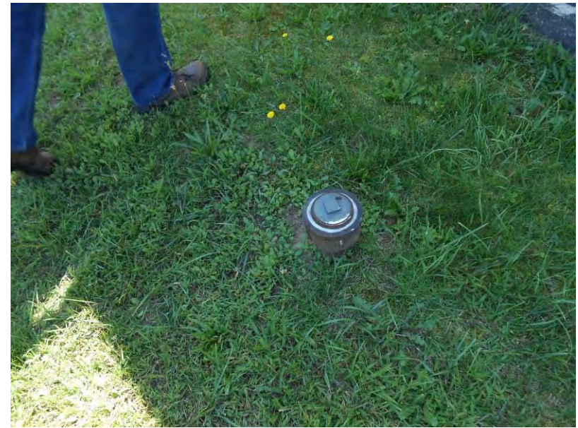
36. View of the potential fill pipe to the suspected UST adjacent to the Lower Building.
