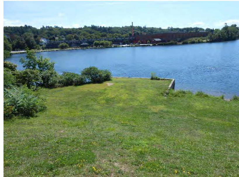
34. View of the foundation of the grist mill looking south.
