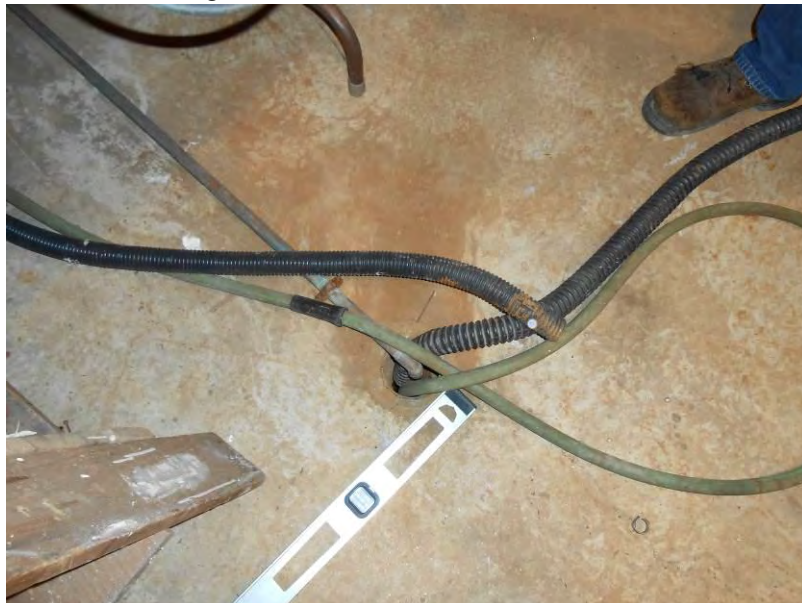
15. View of the floor drain observed in the boiler room of the Madeira office and warehouse building.
