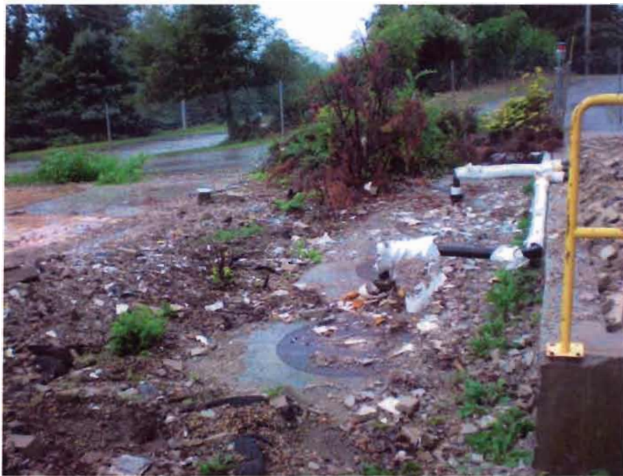
Photo 1 – View of 13,500-gallon UST before removal.
