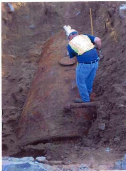
Photo 8 – View of 8,000 gallon-UST uncovered.
