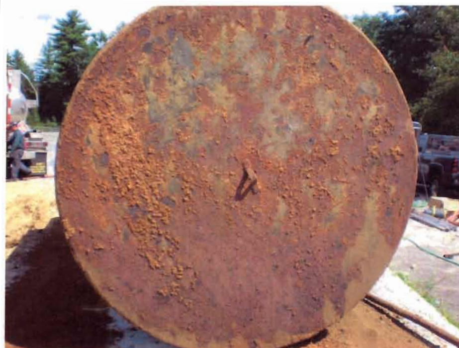
Photo 10 – View of southwestern end of 8,000-gallon UST.
