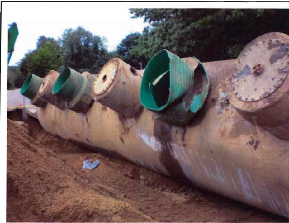
Photo 3 – View of 13,500-gallon UST removed.
