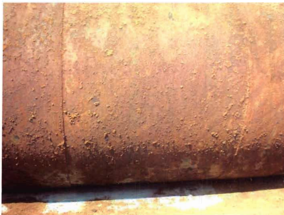
Photo 12 – View of northwestern side of 8,000-gallon UST.
