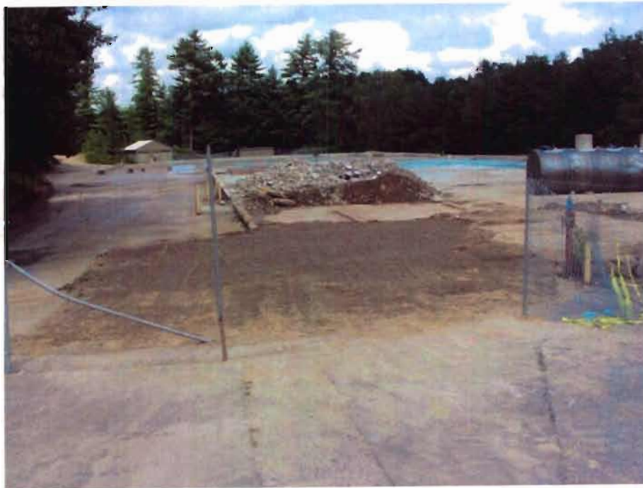
Photo 7 – View of 13,500 gallon-UST basin backfilled.
