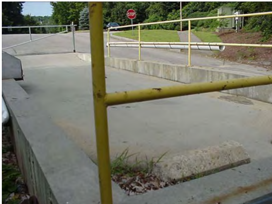
Photo 10 Chemical Loading Dock
