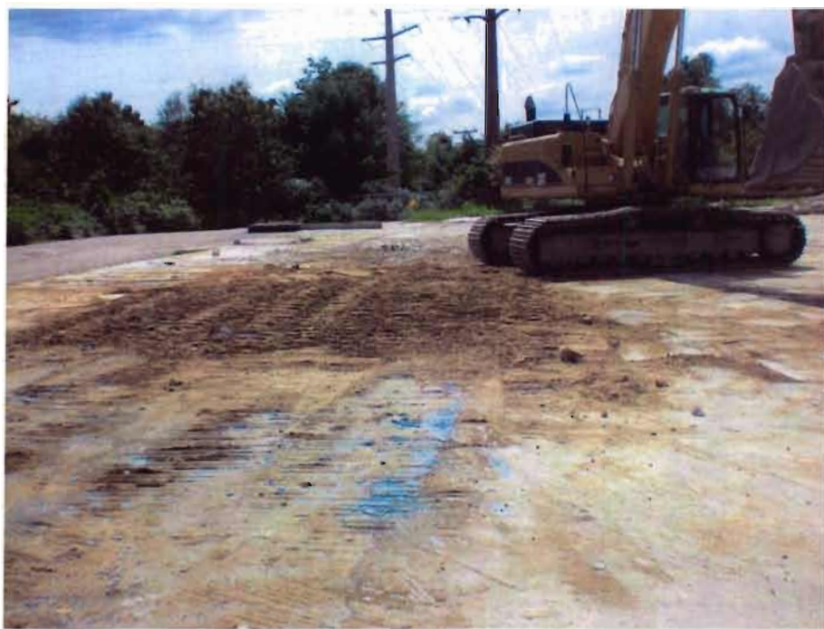
Photo 15 – View of 8,000-gallon UST basin backfilled.
