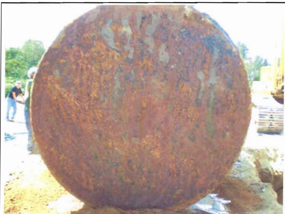
Photo 9 – View of northeastern end of 8,000-gallon UST.
