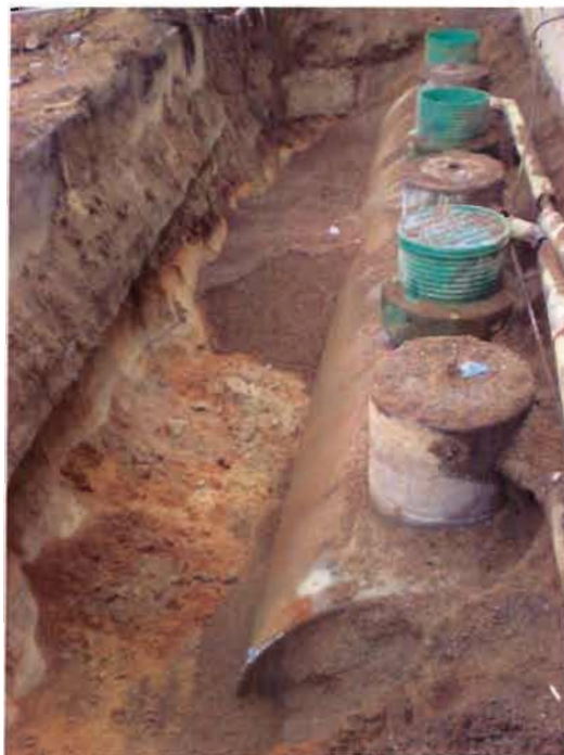
Photo 2 – View of 13,500-gallon UST uncovered.
