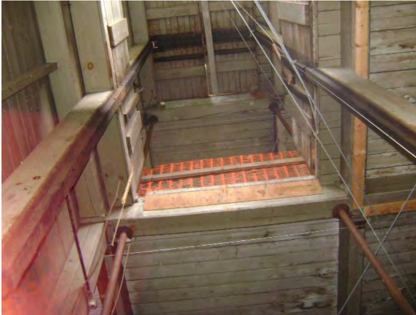
Picture 7 Representative view of the elevator shaft looking up from the first floor.
