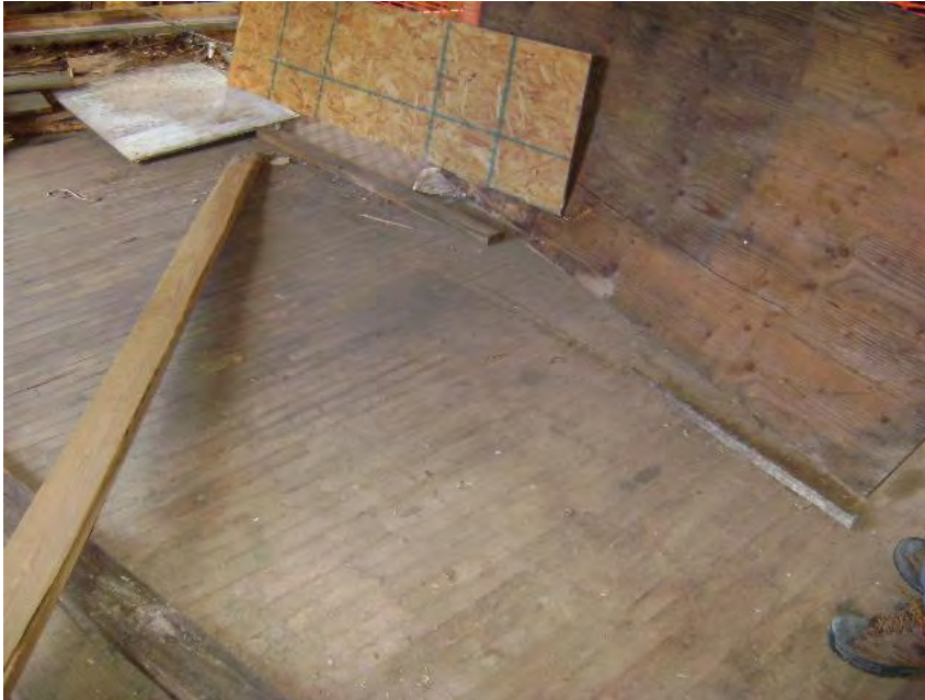
Picture 11 Representative view of wood flooring on all four stories of the building.
