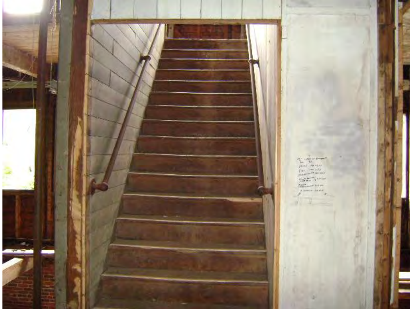
Picture 8 Representative view of the staircase on the first floor.
