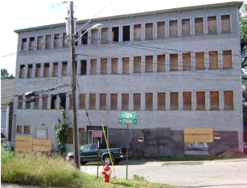
Picture 1 Representative view of the subject property from Spring Street.
