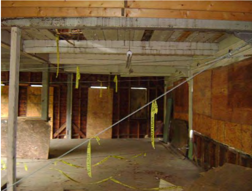
Picture 9 Representative view of the cable bracing supporting the building.
