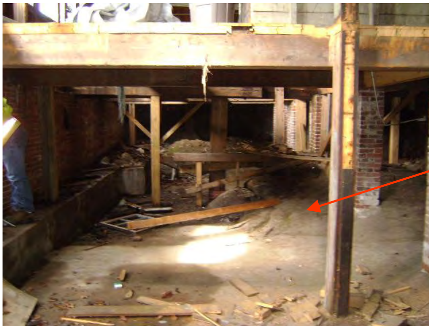
Picture 10 Representative view of the basement looking west.
