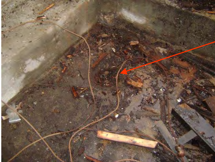
Picture 12 View of the eastern floor drain in the basement.
