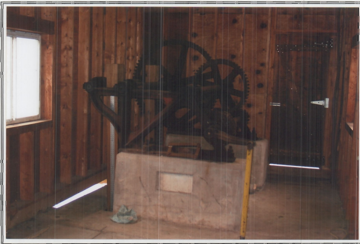
Photo 30. Another interior view of Gate House building showing mechanism for regulating water flow into water powered turbine.
