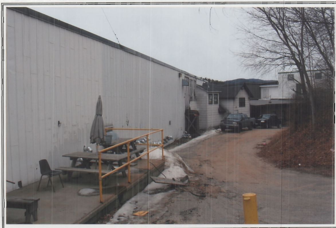
Photo 12. View of connector wing between new yarn plant and wet finish area, roadway to right, looking west.
