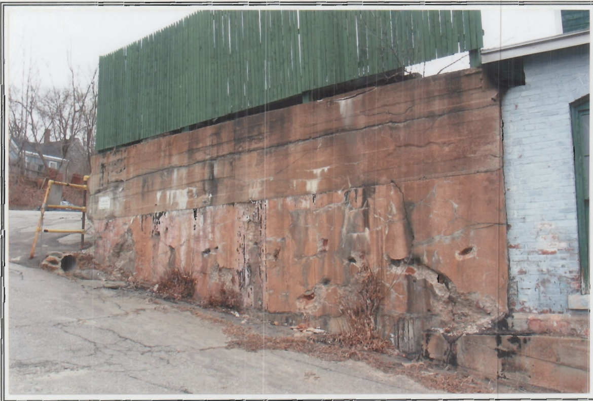
Photo 8. View of concrete retaining wall for former no. 6 fuel oil underground storage tanks, looking north from Hill Street. Mechanic Street in left background.
