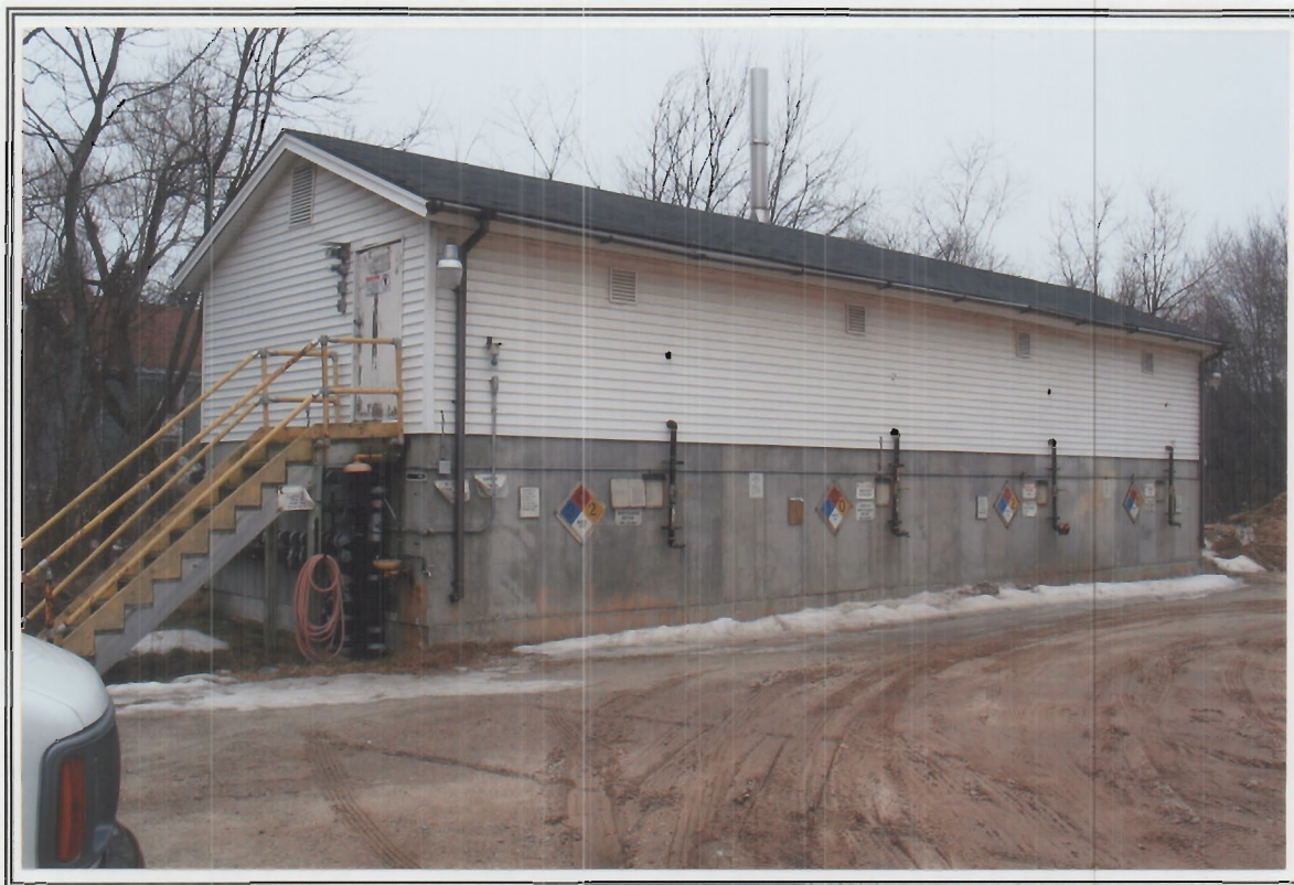
Photo 5. View of north side of bulk chemical storage building looking southwest.
