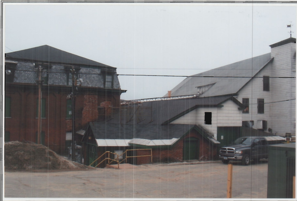
Photo 3. View of northeast side of Scribner Building from Hill Street, looking southwest. White building to right now houses operations of Elpakco Electronics. Outdoor electric power transformer at right bottom of photo.
