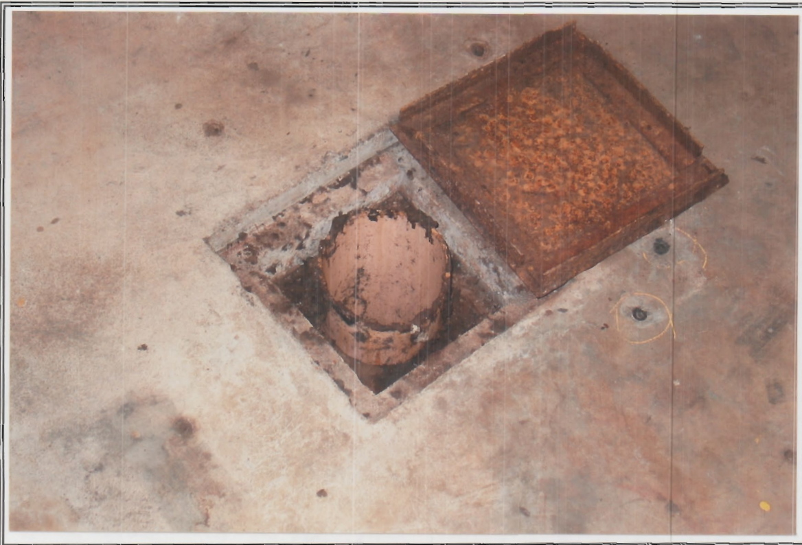
Photo 16. Floor drain, dry finish area within Finishing Department.
