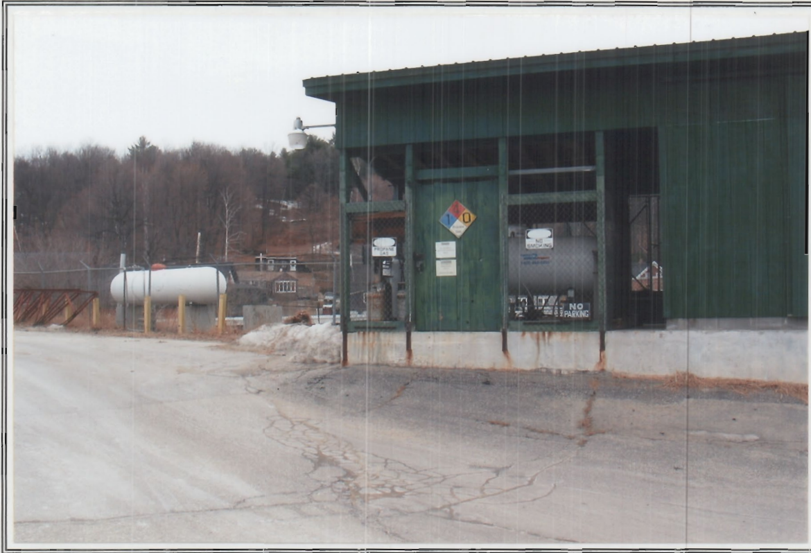
Photo 7. View of propane storage tank area along Mechanic Street.
