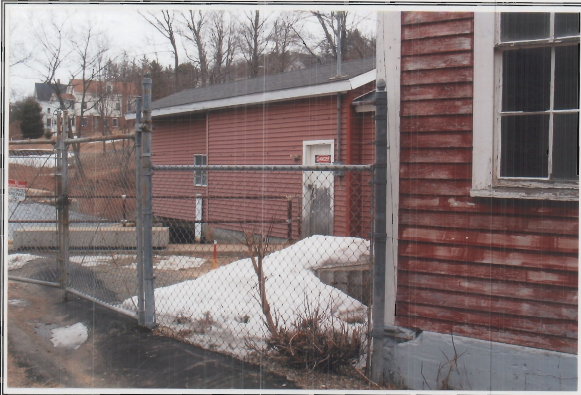
Photo 15. View of gatehouse building.
