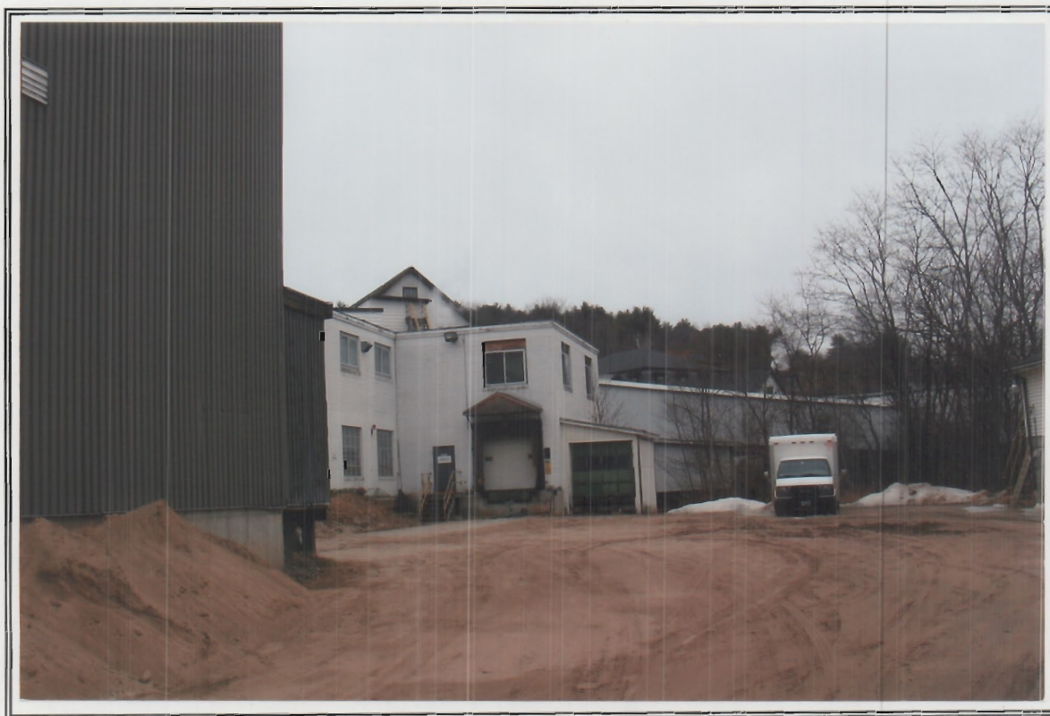
Photo 14. View of south side of new yarn plant to left, looking east. Bulk chemical storage building to far right. Loading dock for Performance Chemicals in center.
