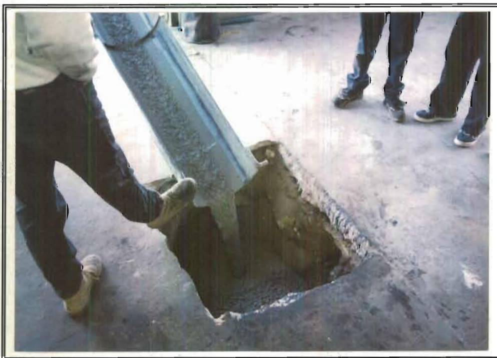
2. Closure-In-Place with Concrete
