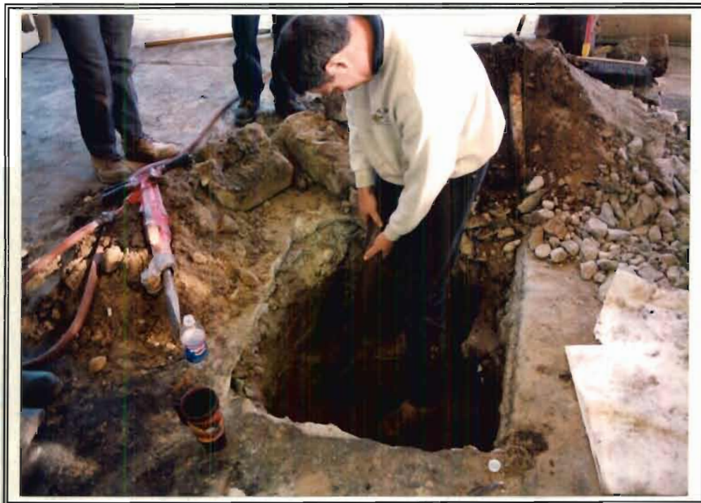
1. Product Removal 500-Gallon Waste Oil UST
