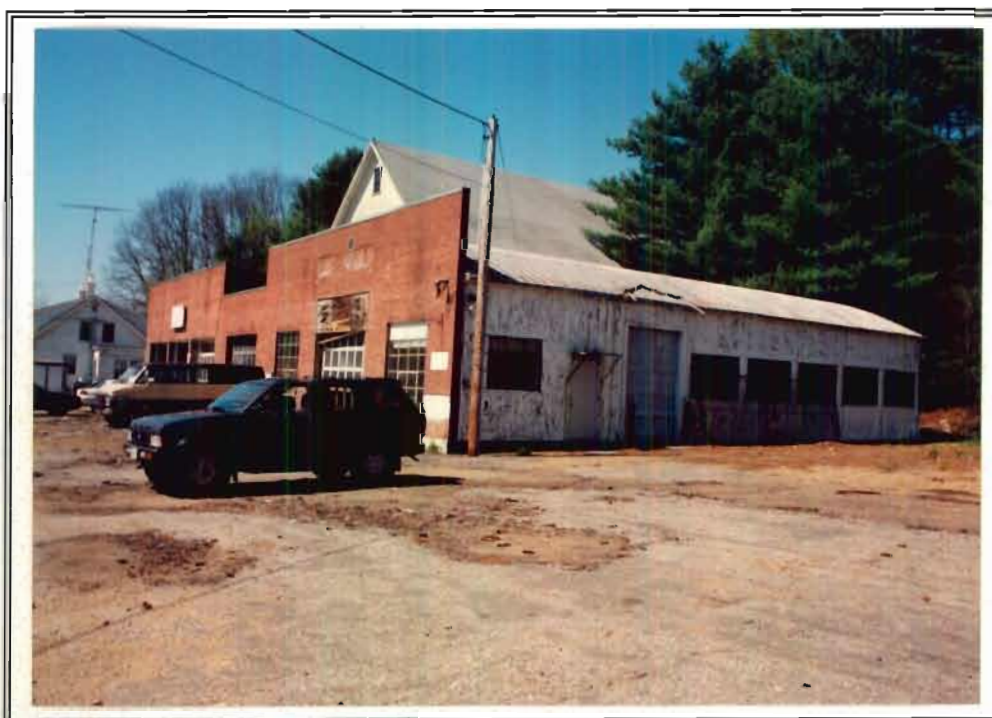
2. Subject Building, North Face Residence at Left
