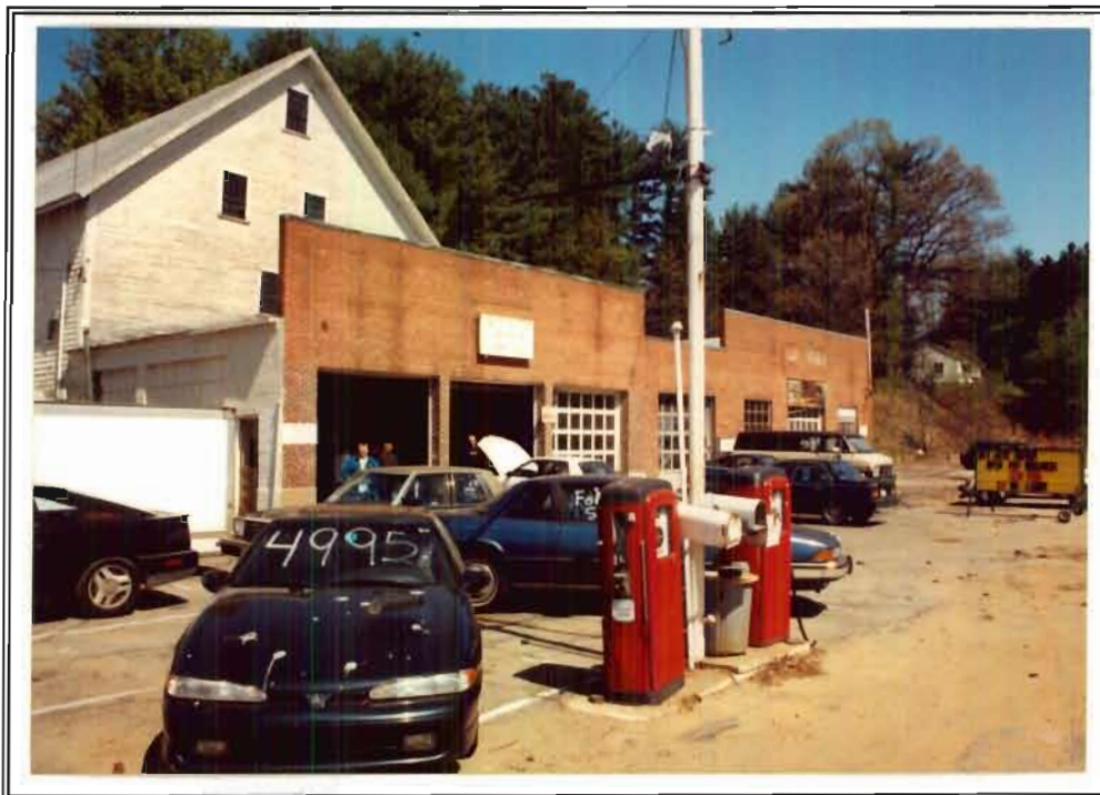
1. Subject Building & Former Fuel Pumps L to R: Barn, Service Garage, Warehouse
