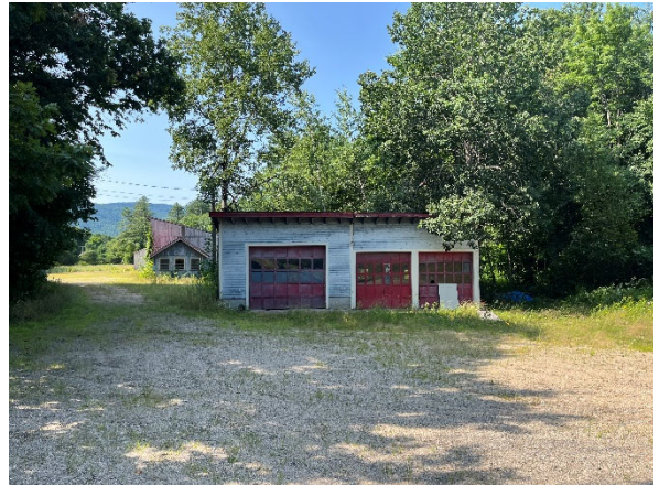
Photo 2: View of three bay garage
