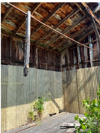
Photo 9: Interior of dipping basin shed
