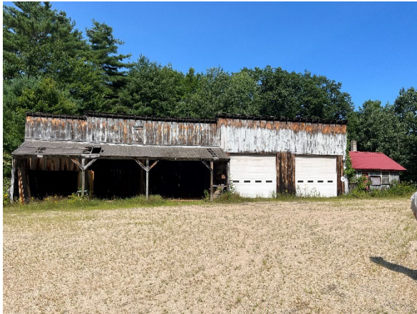
Photo 1: View of open-front garage, two bay garage, and office building
