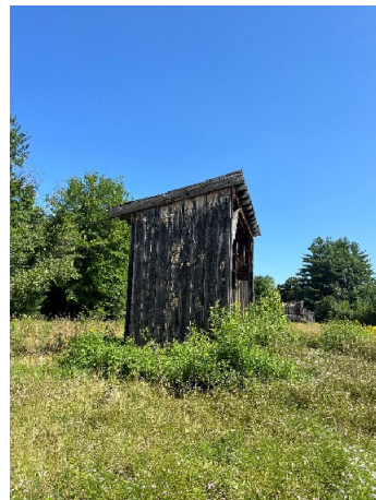
Photo 8: Exterior of dipping basin shed
