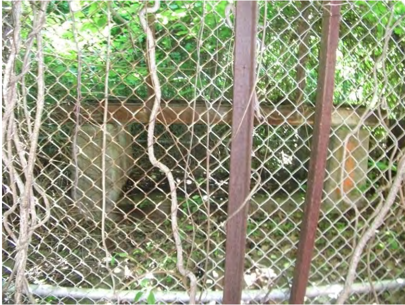
45. Former transformer area outside the northeast corner of the Stanley Mill.
