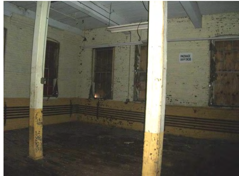
10. Large room in southern portion of the Stanley Mill, first floor.
