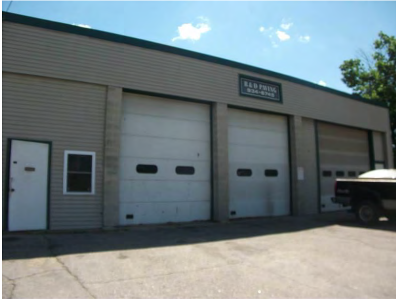
5. Nearby property to the southeast (81 Memorial Street).
