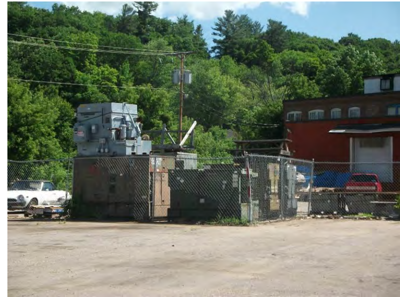
4. Adjoining property to the east (20 Canal Street) looking northeast.
