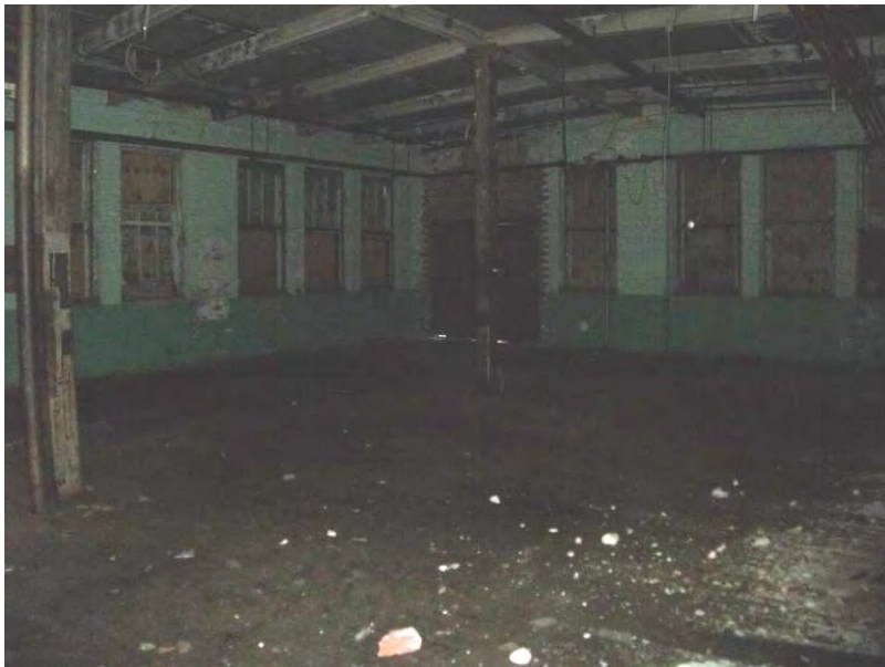
11. Large room in southern portion of the Stanley Mill, first floor.
