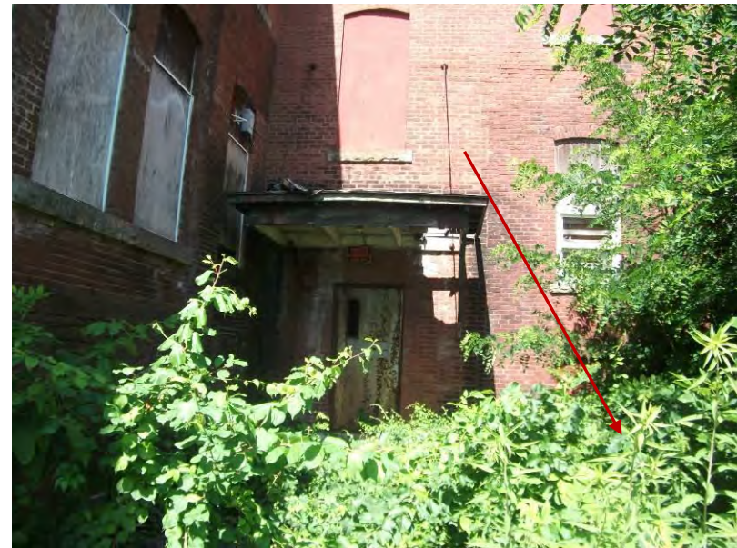
52. Location of former 10,000-gallon fuel oil UST at the Stanley Mill. Note the dense vegetation.
