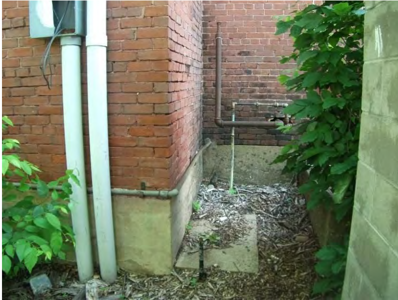
41. Concrete pads near northwestern corner of the Stanley Mill.
