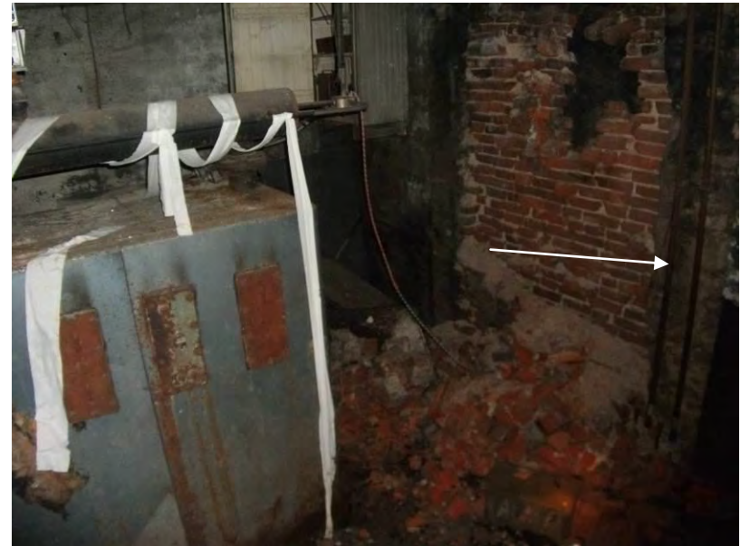
22. Location of fuel lines on northern wall of boiler room of Stanley Mill.
