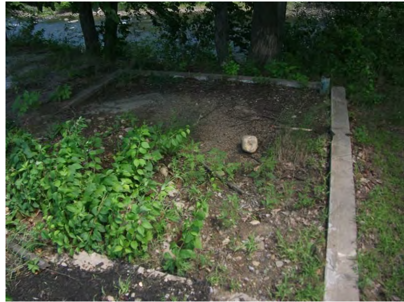
40. Foundation near northwest corner of former Armory.
