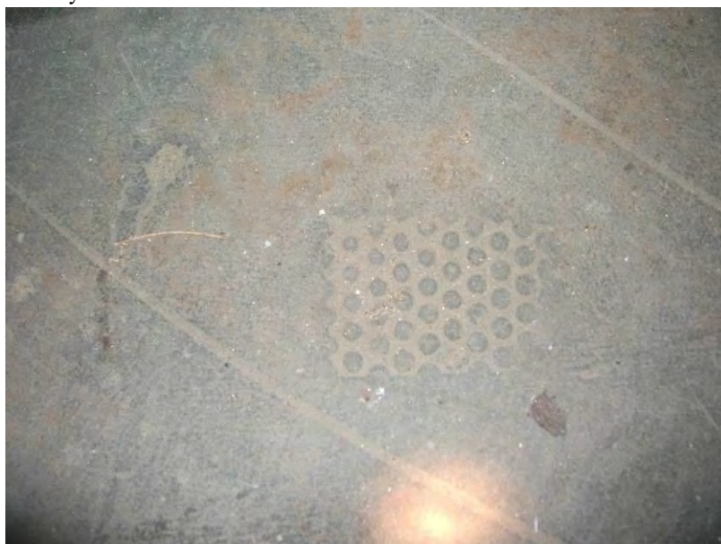
31. Rubberized coating on floor of former Armory.
