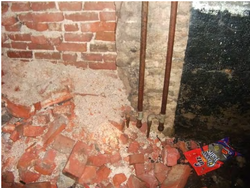
23. Location of fuel lines on northern wall of boiler room of Stanley Mill.
