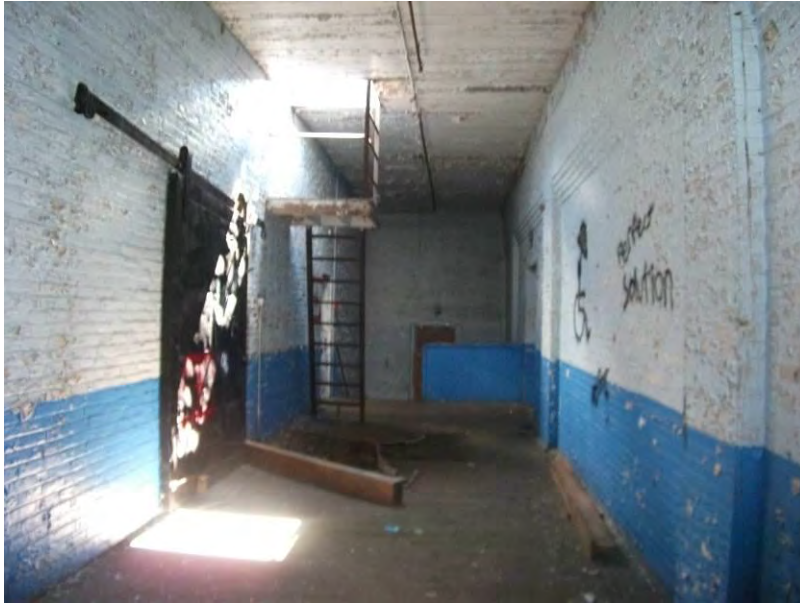
17. Location of roof access in hallway of second floor of the Stanley Mill.
