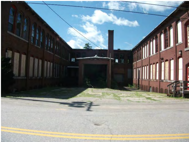
7. Adjoining property to the south (100 Memorial Street) looking south.
