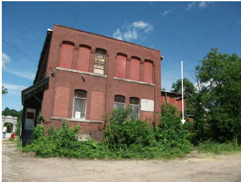
51. Location of former 10,000-gallon fuel oil UST at the Stanley Mill.
