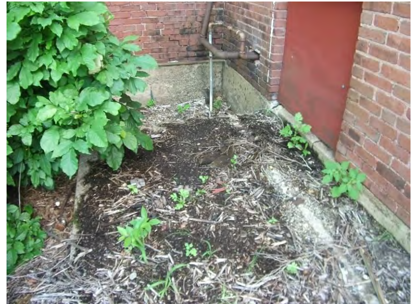
42. Concrete pads near northwestern corner of the Stanley Mill.
