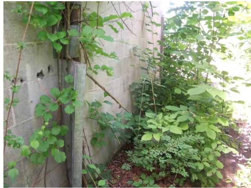
48. Fill and vent pipes on northwest corner of the former Armory.
