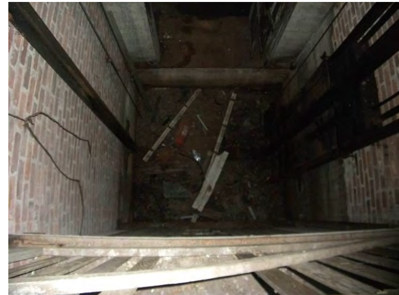
16. Elevator pit in southwest portion of the Stanley Mill.
