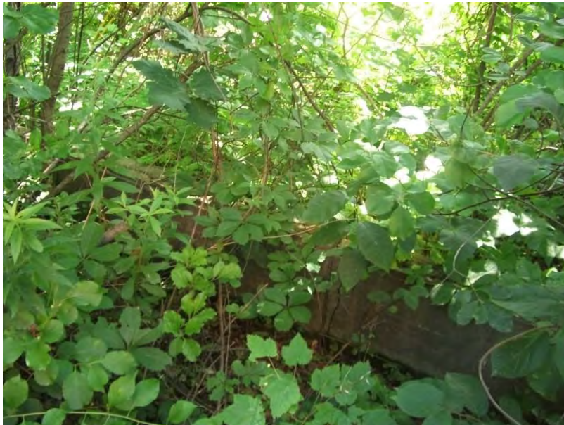
39. Foundation of former garage east of the Stanley Mill.
