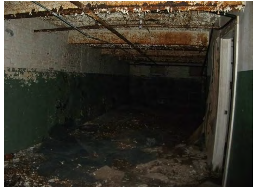
18. Conditions in basement of Stanley Mill.
