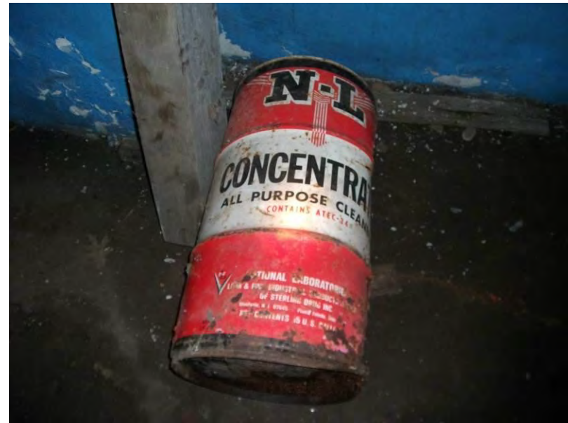
20. Discarded drum of cleaner concentrate in basement of the Stanley Mill.
