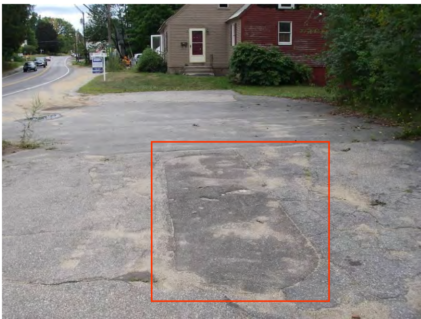
Picture 4 View of pavement patch where former fueling island was located.
