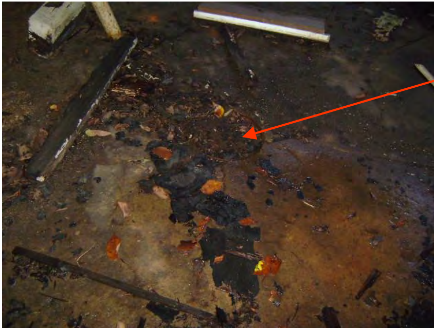
Picture 17 View of the floor drain in the garage bay.
