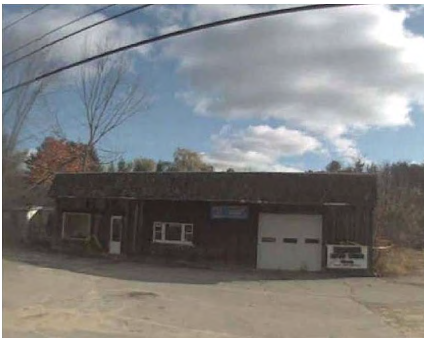
Picture 1 Representative view of the subject property from East Main Street.
