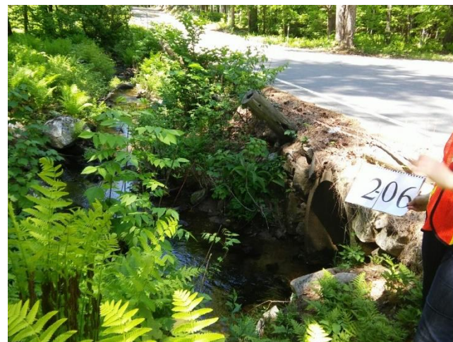
Site 2-06: Rt. 113 at Transfer Station Rd (Burrows Brook).
