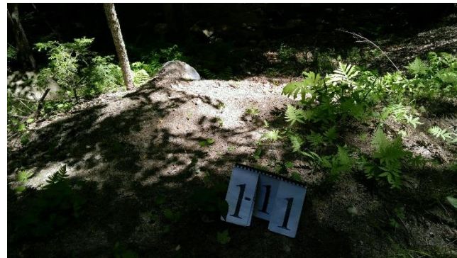
Site 1-11: Stormwater outfall pipe from Owl Brook Rd.
