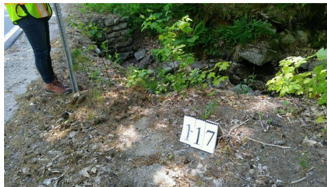
Site 1-17: Road crossing on Rt. 113 (West Brook).
